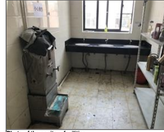
Photo of the sanitary facilities 131 Drinkable water.JPG
